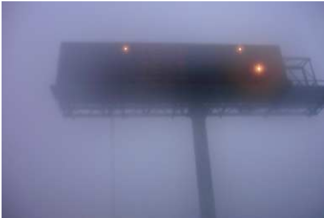
Figure 2.9.1.3. Photograph of CMS during very poor visibility. The message displayed on the CMS is “TEST TEST TEST”.
